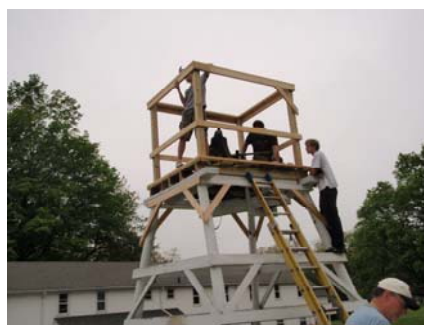
New Bell Tower Roof Construction
